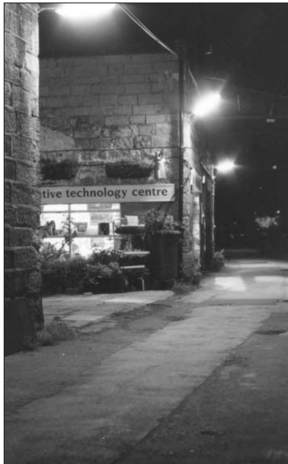
Solar powered street lighting outside the ATC. The three street lights now installed outside the ATC at Hebble End run off electricity generated by sunlight. During the day, two 64 watt photovoltaic panels generate electricity which is stored in batteries inside the Green
