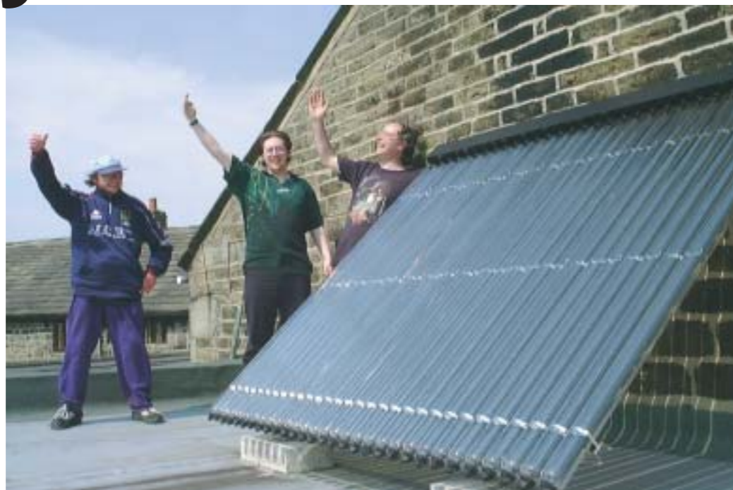
Nick Wilding, pictured here with his sons Gabriel and George, installed solar water heating last year at his home in Heptonstall.
